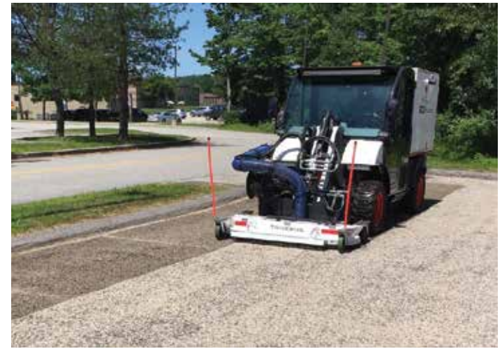
A Triverus MCV cleaning pervious asphalt at UNHSC
